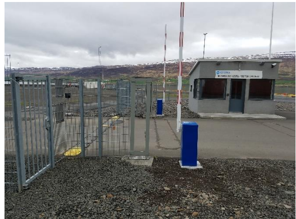
Picture 2-2: Measurements at the main entrance gate
